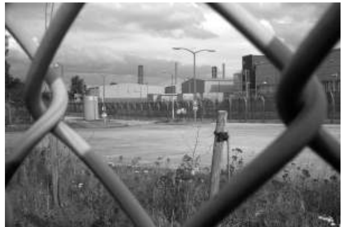
Medium level waste is stored in these buildings
